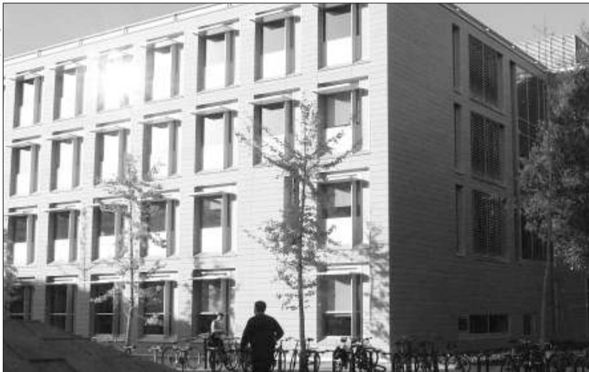
The new English Faculty building: the latest in a centuries-old tradition of dark, subversive architecture
